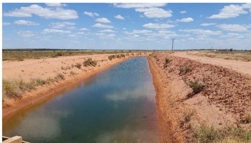
Figure 5: Main irrigation canal of the Formoso River, below grade from agricultural fields.
